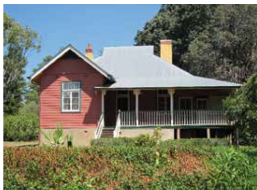
The heritage-listed Constable's Cottage built in 1913 still stands as a reminder of a police presence around the formative Canberra community.
